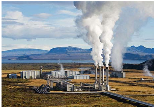
Figure C-6: A geothermal power installation
