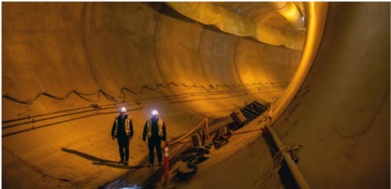
Figure 24: Diversion Tunnel, Site C Dam, Fort St. John
